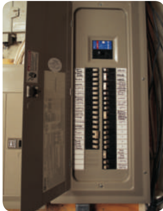
This circuit breaker box (right) controls a home's circuits.
