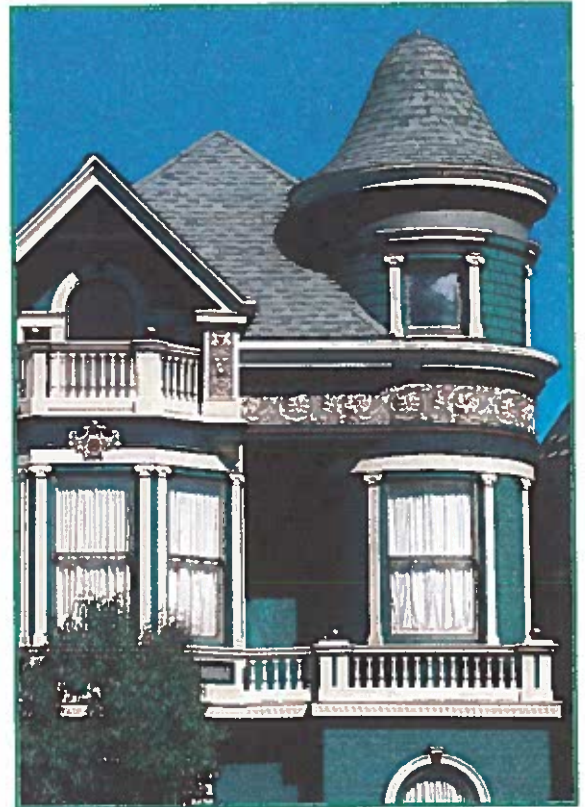
▲ This roof is built with shingles. The shingles are small flat pieces of slate.
