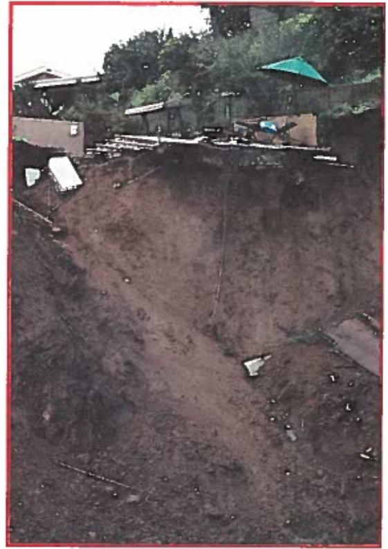
▲ Homes in the Los Angeles, California area damaged by mudslides
