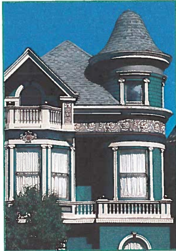
▲ This roof is built with shingles. The shingles are small flat pieces of slate.
