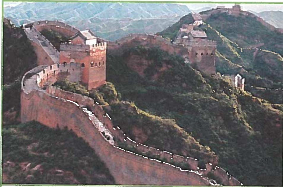
The Great Wall of China was made from blocks of granite. It was built over 2,000 years ago.
